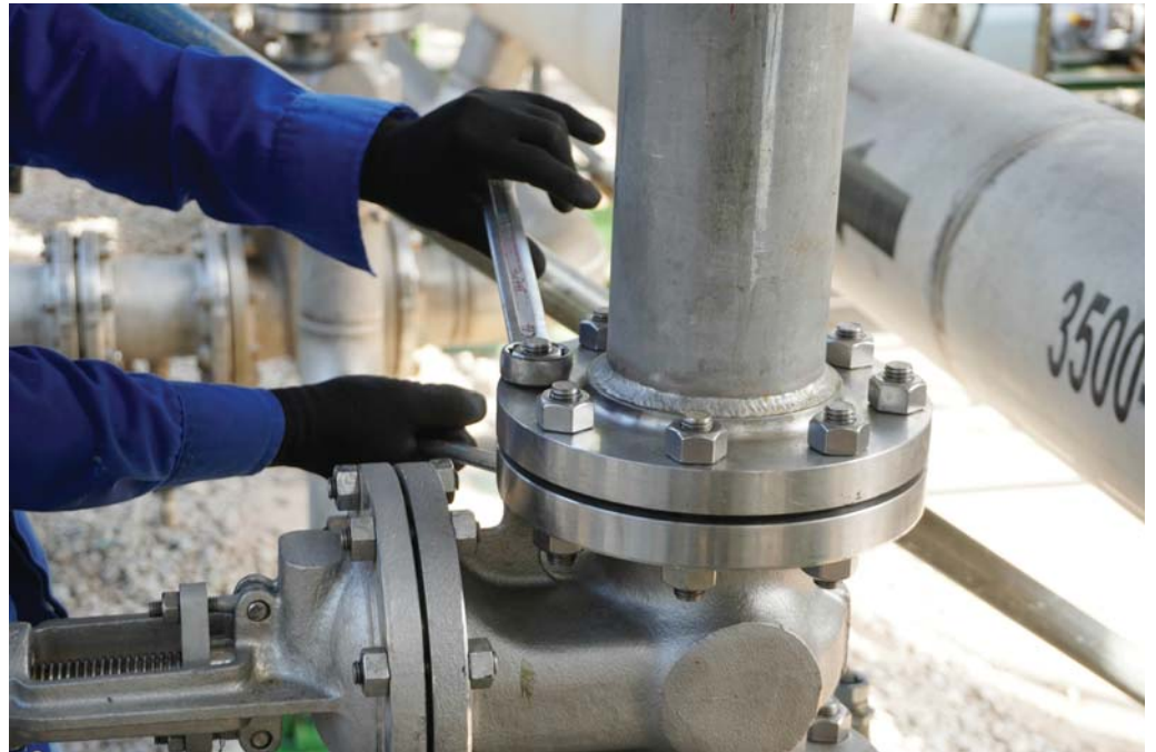
Gasket guess work; no torque indication.
